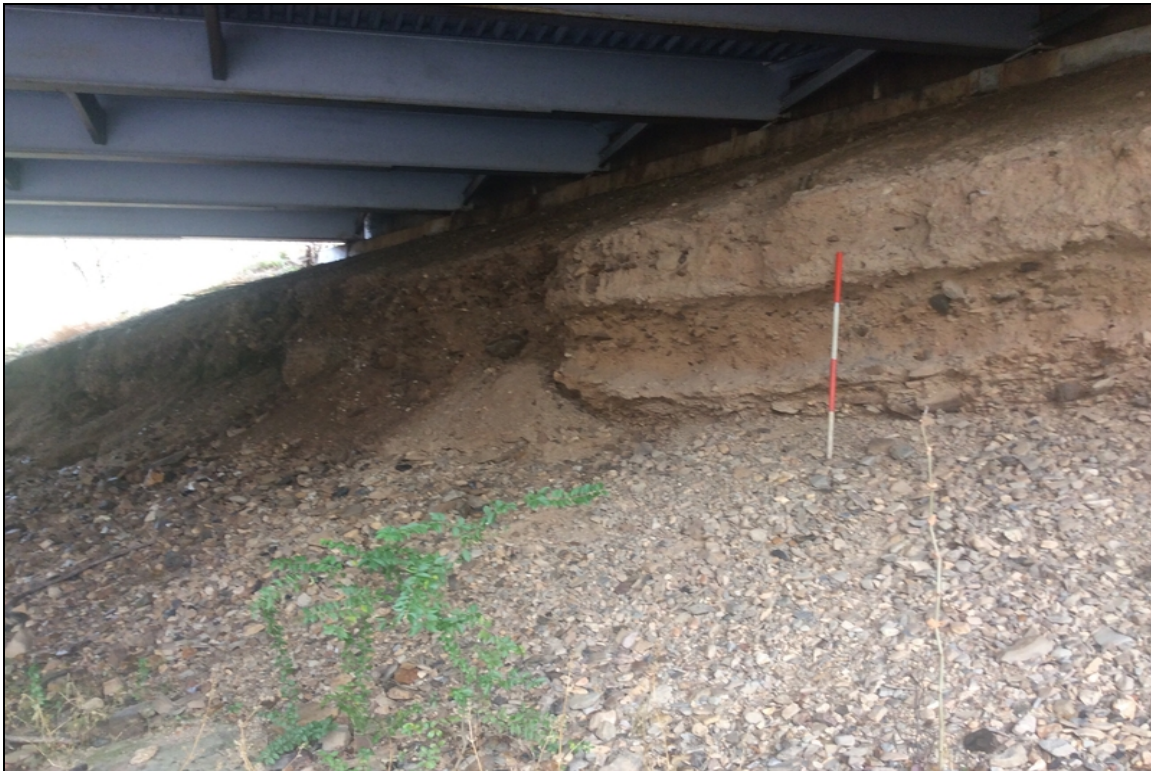
Bent 4 embankment erosion.
