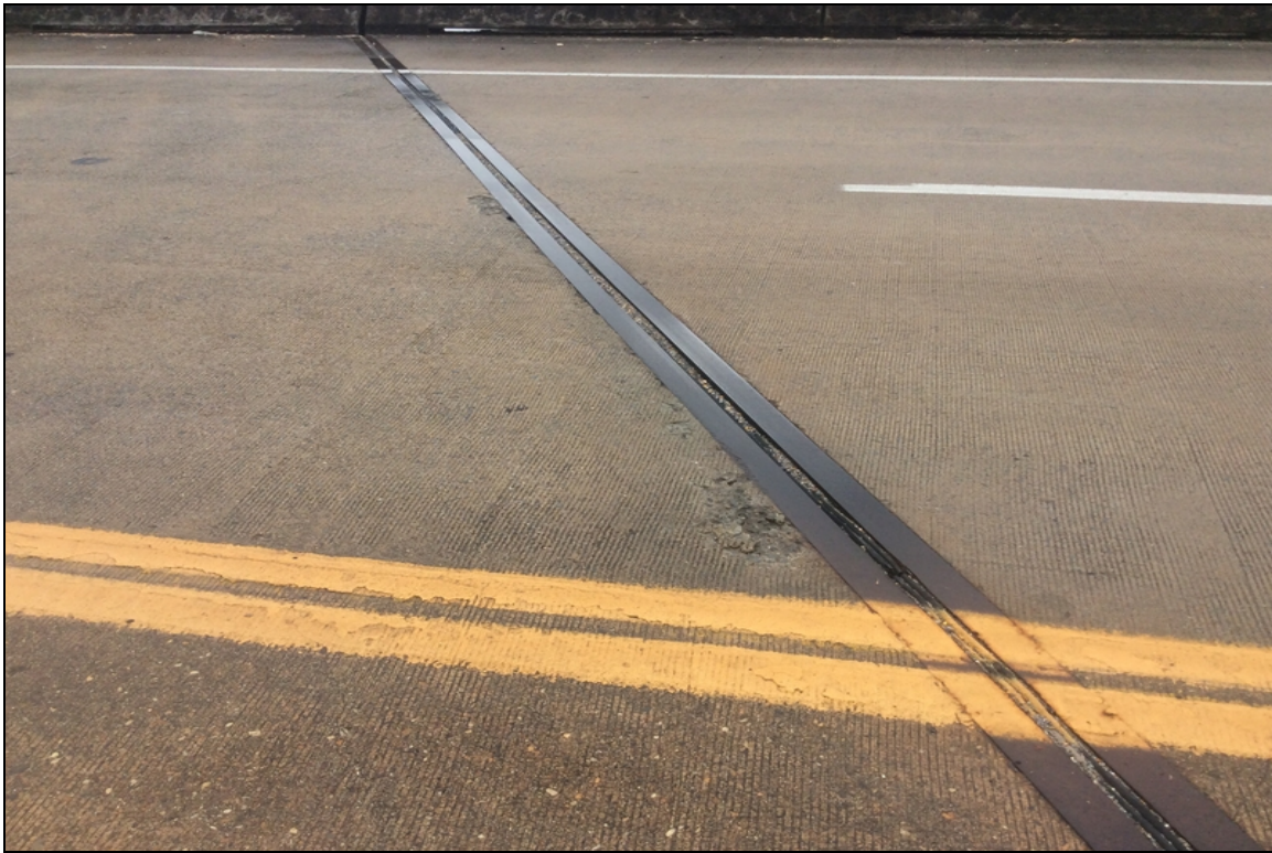
Large spalls in span 3 near bent 3 joint eastbound lanes.
