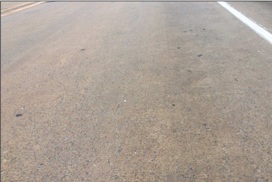
Span 1, longitudinal cracks.
