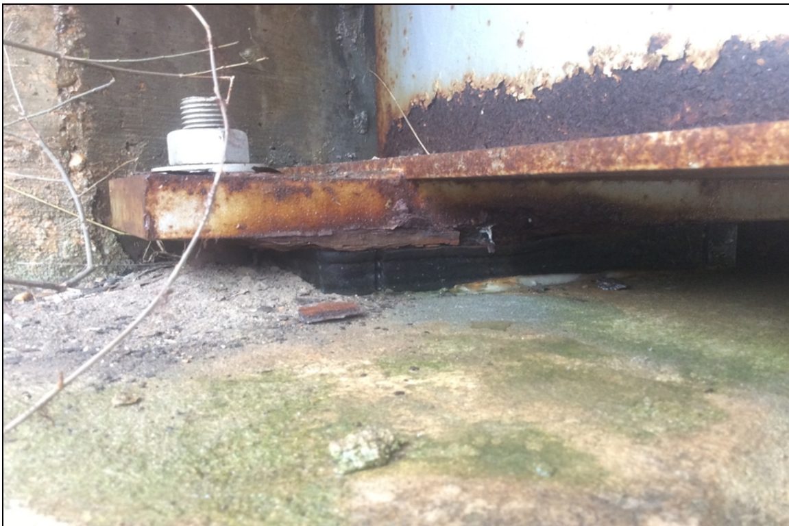
Bent 4 bearing 1, severe corrosion on the sole plate.
