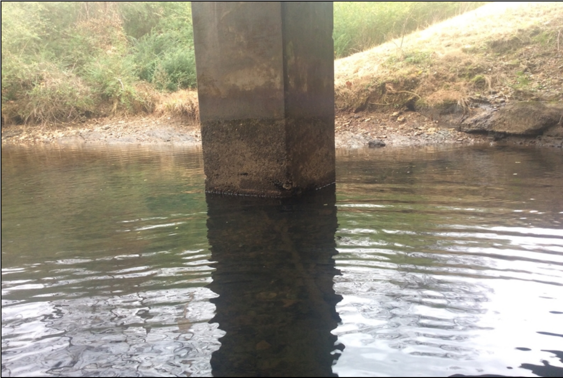
Bent 3 column 1, severe abrasion.
