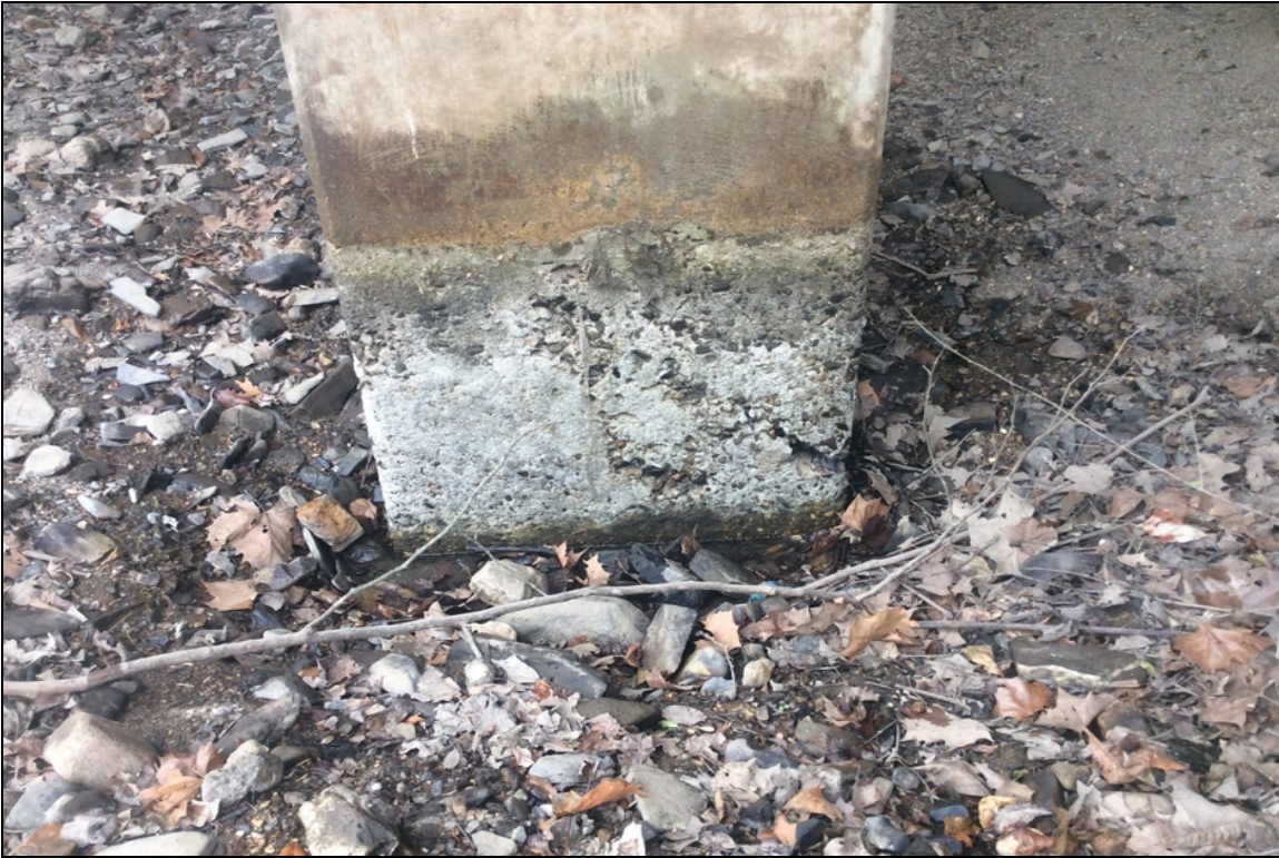
Bent 3 column 1, severe abrasion.
