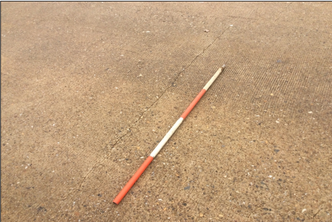
Large transverse crack in Span 3.
