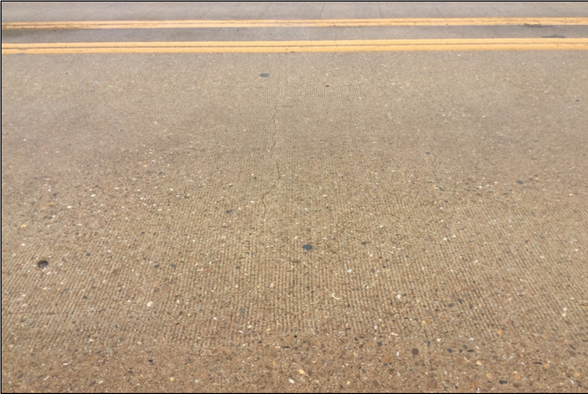
Transverse crack Span 1.
