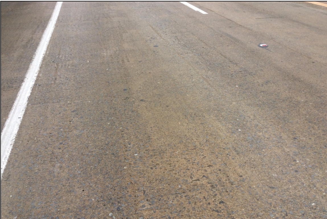
Span 3, abrasion
