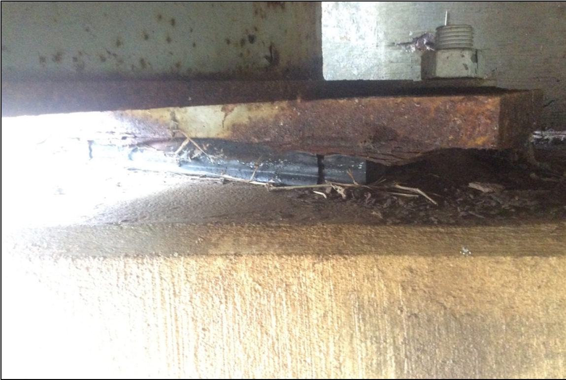
Bent 1 bearing 10, severe corrosion to sole plate.
