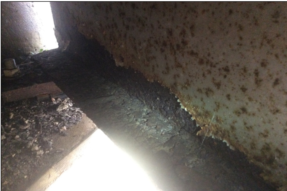
Bent 4 beam 10, corrosion with section loss to bottom flange and lower web.
