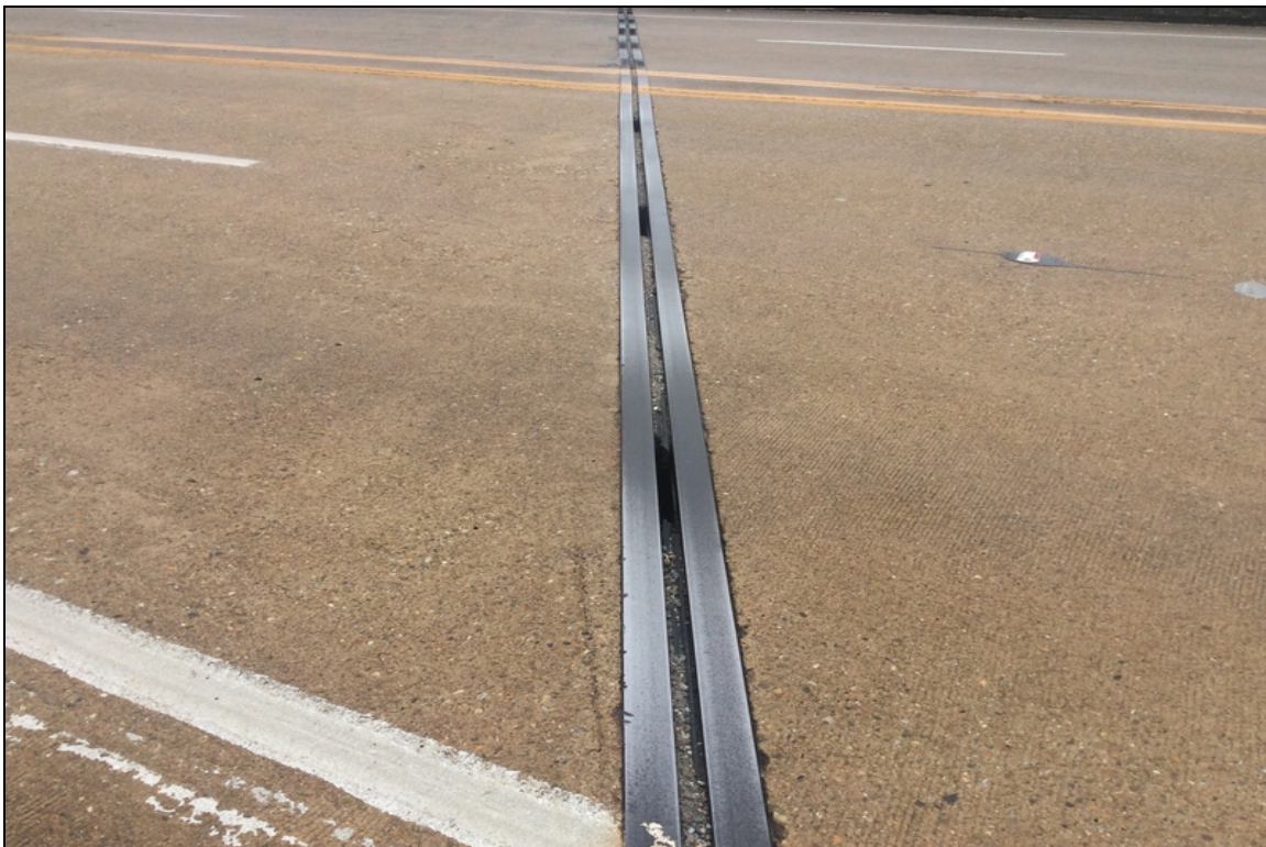
Bent 3, joint is missing in three areas of the westbound lanes.
